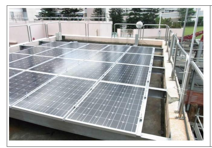
2,800W solar photovoltaic panel system 太陽能光伏板-2,800W
